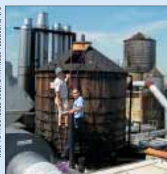
Physicists convert a water tank at New York University to detect particles from space.
